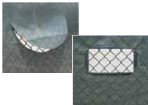
Half-moon air vents or 6" x 12" boxed air vent
