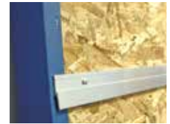
Additional Z-clip mounting attachments. Easy removal, repair or replacement of wall panels (no nail margins).
