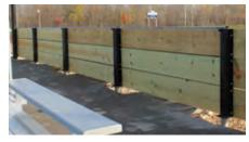
**Slide-over post brackets** are added over wall posts and pressure treated wood planks are mounted to custom hardware.
