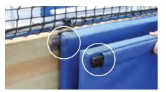
Full-length **support battens** hang on the mounting brackets and the bottom edge of the pads is secured to Velcro.
