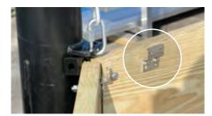
Stainless steel **mounting brackets** and **Velcro wall plates** are added in preparation for adding Wood-less Pads.
